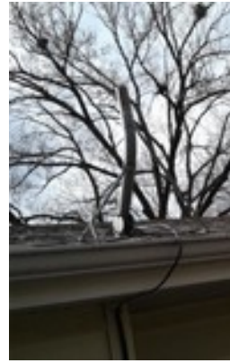
Figure 15: Old TV Satellite mount adjusted so pole points up.
