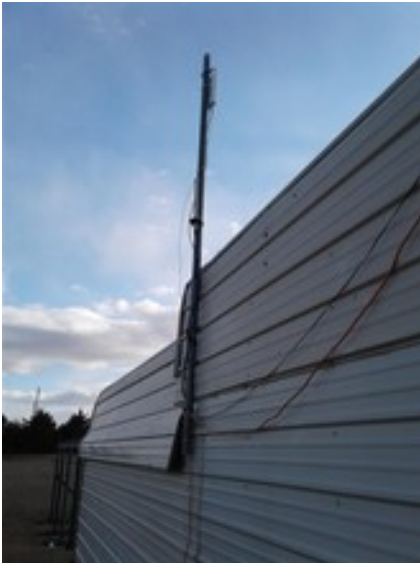
Figure 17: Pole along wall with no over hang.
